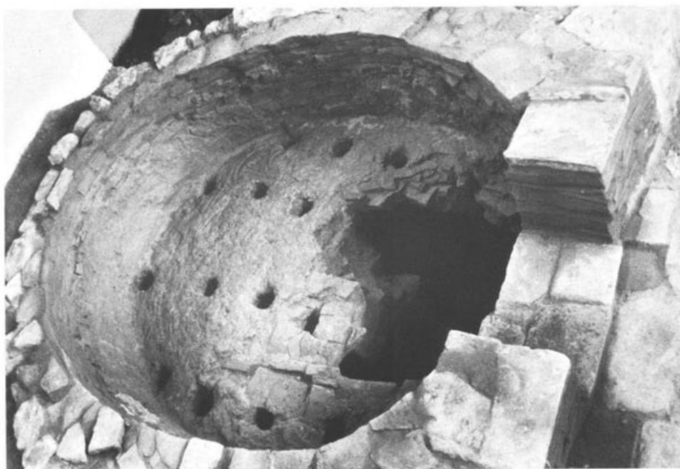
Foto 4. Kiln II Top view showing the ware chamber and remaining portion of the pierced floor.
